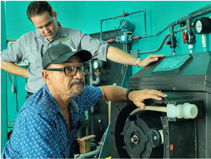
Hip and Igor discovered the problem was related to an installation error. The initial problem was quickly rectified, and the pump was running smoothly. A second pump had yet to be installed and before installation of the second unit began, Igor and Hip conducted training for the operators. Then, stepped back and watched as the gentleman installed the pump. If an error was made, the operator was stopped long enough for Hip and Igor to discuss and demonstrate the correct procedure.
